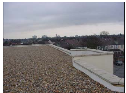
Roof and parapet wall
